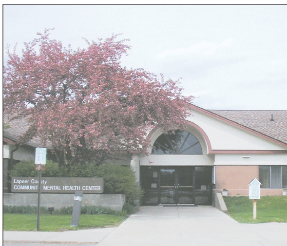
Lapeer County CMH main office.
